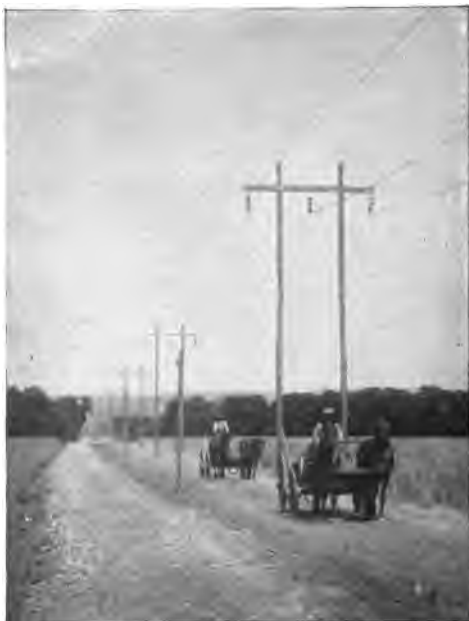
FIG. 239. The three-phase three-wire line from Meppen, Ill., to Alton, Ill. The General Electric Review.
